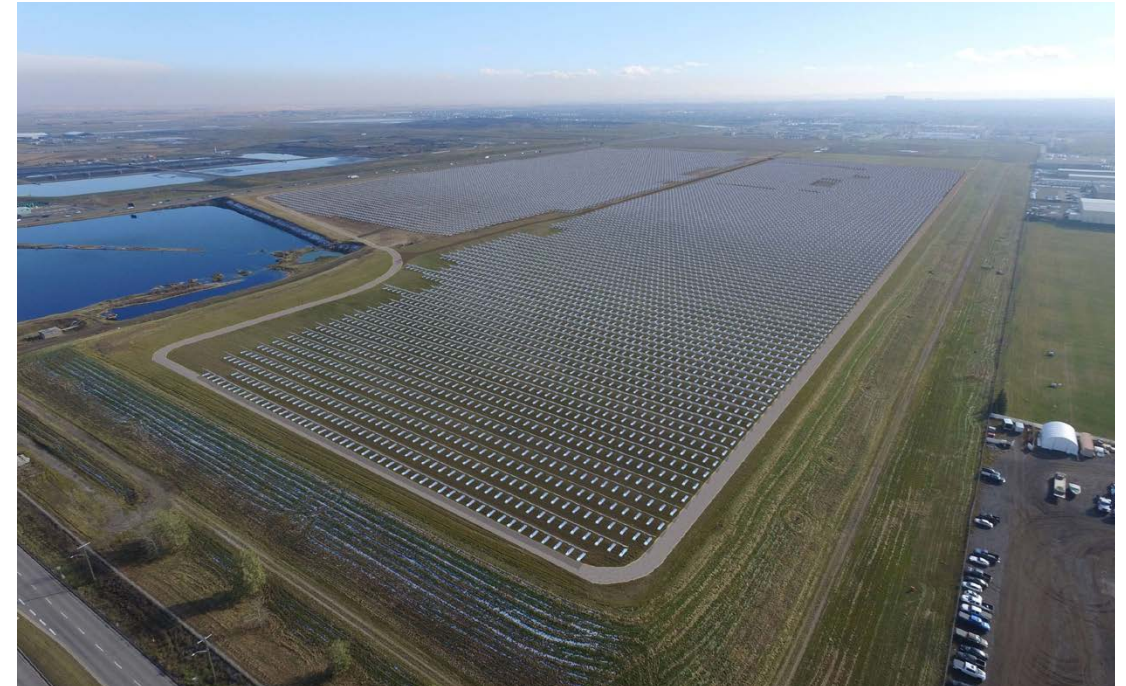
We use bifacial panels at our Barlow and Deerfoot solar projects to generate electricity from both the direct sun on the front face and the reflected sun on the back.
