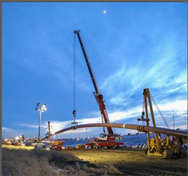
NATURAL GAS TRANSMISSION
