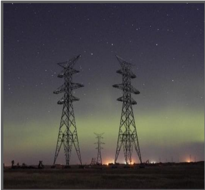
FORT MCMURRAY WEST 500 KV TRANSMISSION
