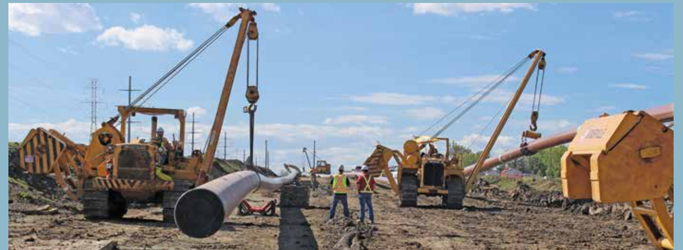
Through the UPR Program, ATCO Pipelines is building new, high pressure pipelines in Transportation/Utility Corridors in Calgary and Edmonton.
