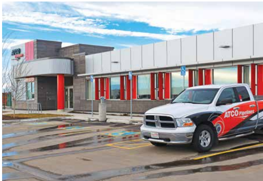
In December 2015, ATCO Pipelines opened its new 19,000 sq. ft. South Operations Centre in Airdrie. It features 12,000 sq. ft. of office space, room for material and equipment storage, and two drive-through vehicle bays and a storage bay.
