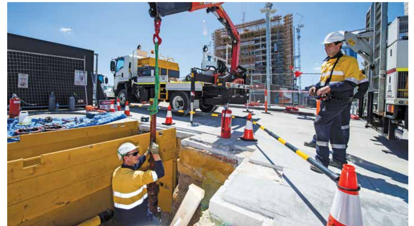
Nick Smith and Aden Bourke, Gas Distribution Officers, commissioning a new gas main pipeline to Kings Square in the Perth city centre, part of one of Australia's most significant urban renewal developments.
