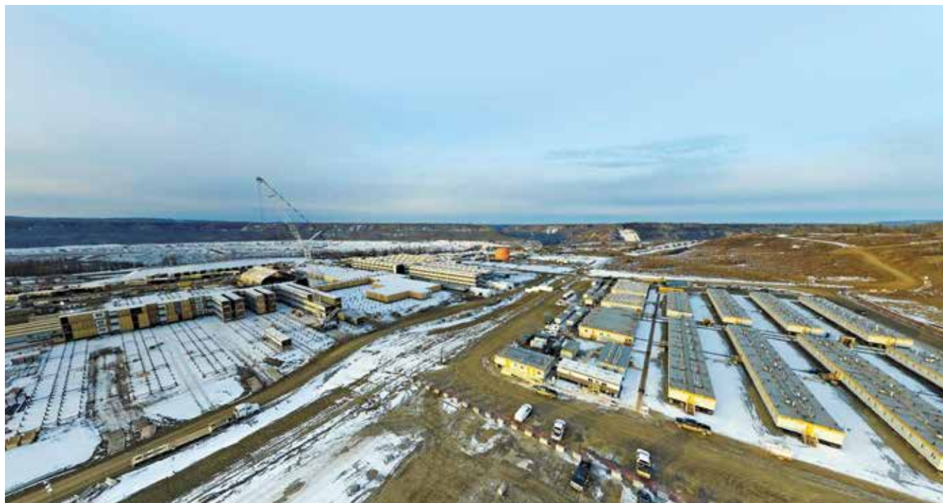
ATCO Structures & Logistics is building a temporary community in the form of a 1,600-person workforce housing facility for the construction of BC Hydro's Site C Clean Energy Project.
