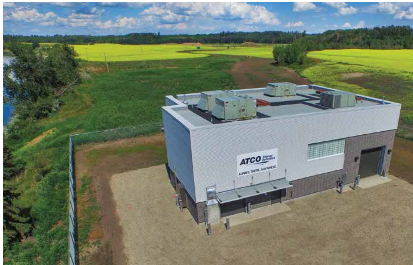
ATCO Energy Solutions' new industrial water pump station, strategically located on the North Saskatchewan river in Alberta's Industrial Heartland.
