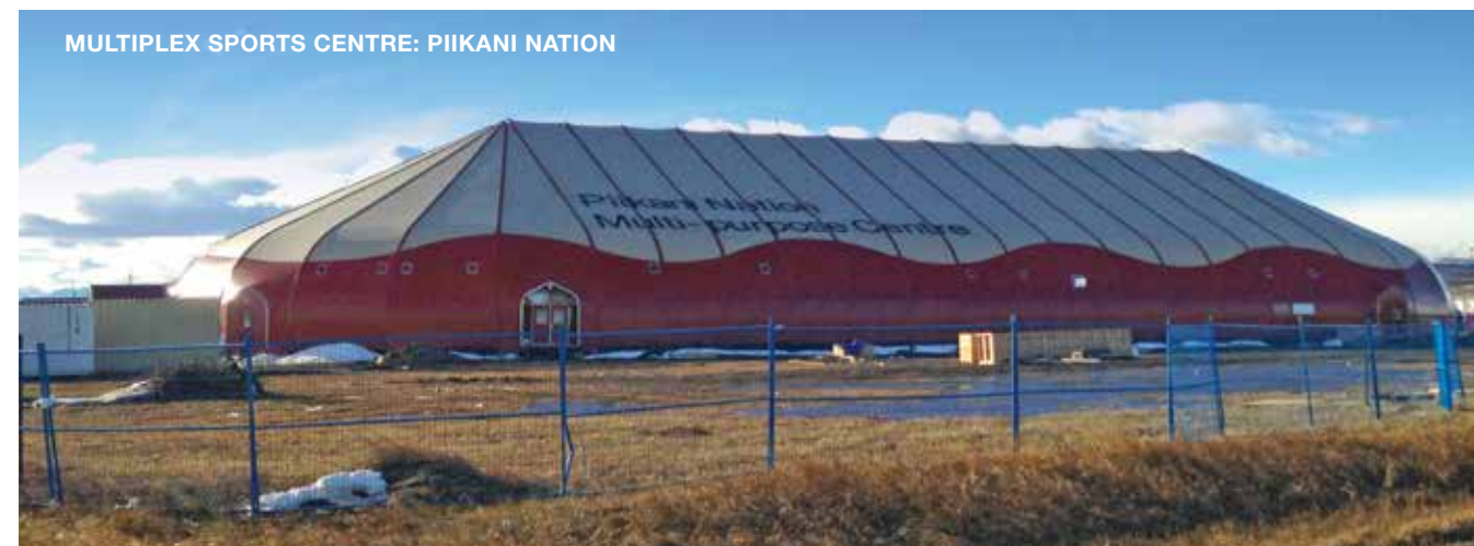
When complete, the Piikani Nation's state-of-the-art 36,000 sq. ft. multiplex sports centre will be the largest project in ATCO Sustainable Communities' history.
