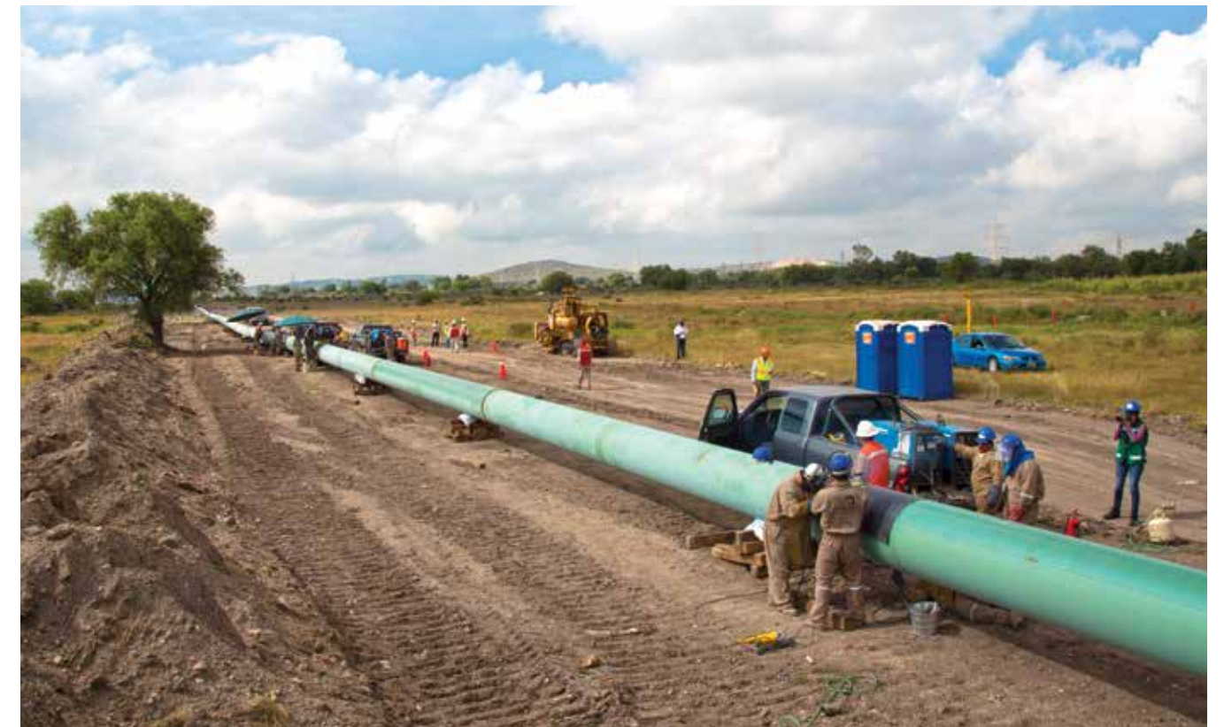
Construction on ATCO's Ramal Tula Gas Pipeline is well underway. The pipeline will transport natural gas to the Comisión Federal de Electricidad's Francisco Pérez Ríos thermoelectric power plant.
