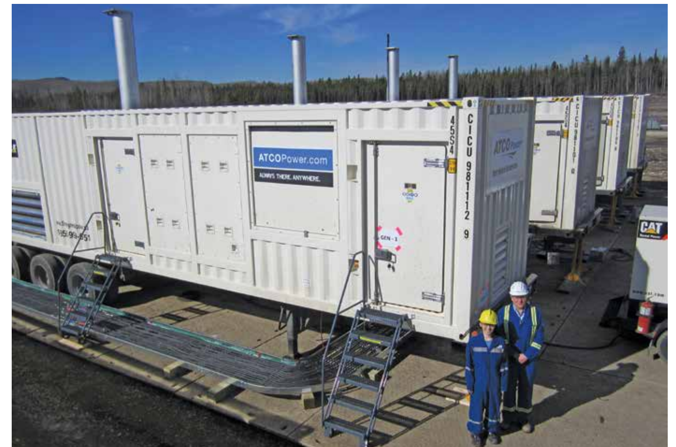
ATCO Power's Distributed Generation team successfully delivered a 5 MW temporary power generation solution that reduces flare gas for Apache Canada Limited. Temporary power solutions can be used to bridge the gap between grid connection and permanent generation for emergency or supplementary onsite power or to offset electricity shortages.
