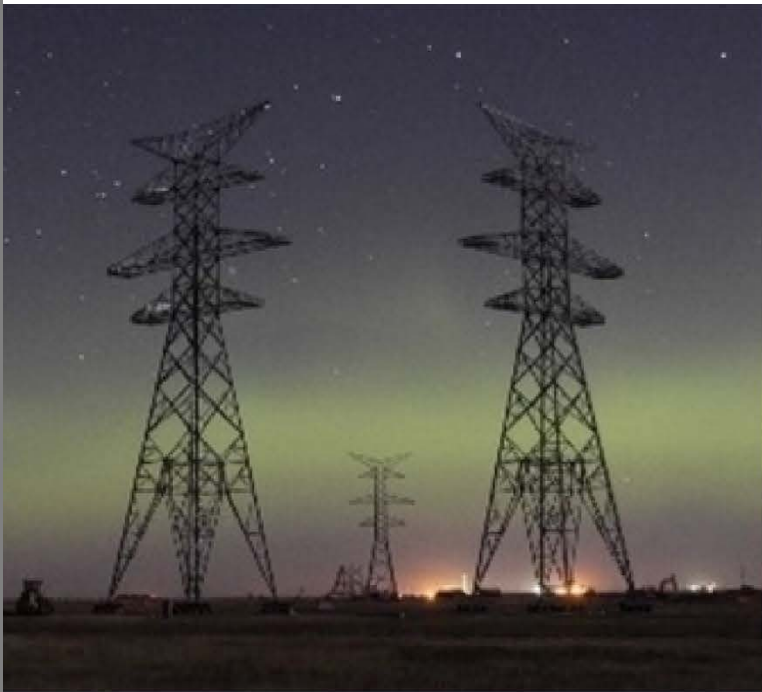
Fort McMurray West 500 kV Transmission
