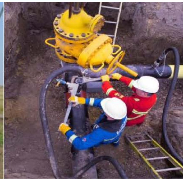
Natural Gas Transmission
