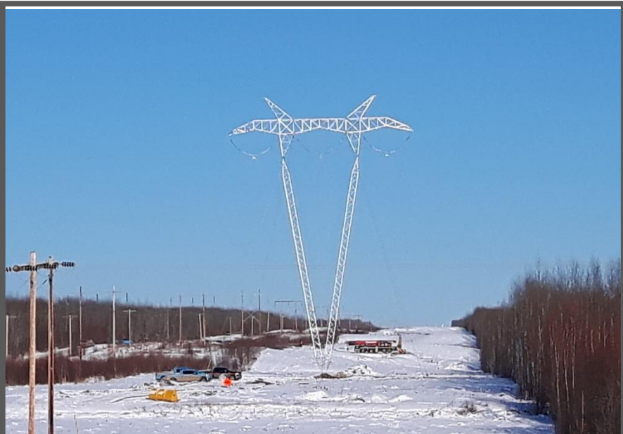
FORT MCMURRAY WEST 500 KV TRANSMISSION
