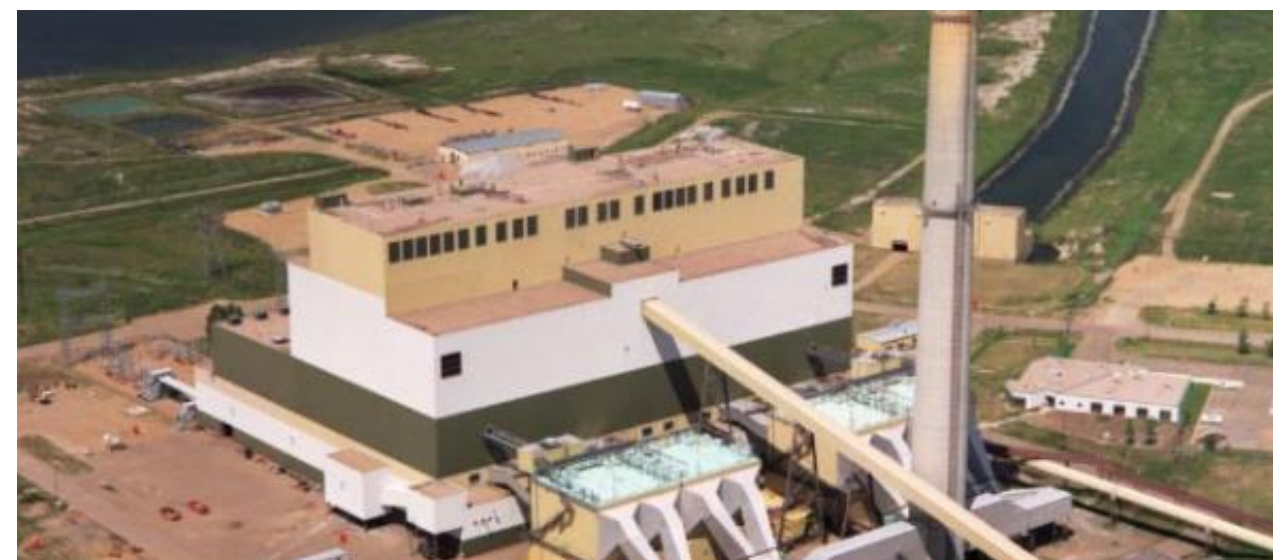
Sheerness Generating Station
