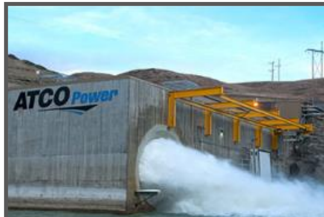
ELECTRICITY GENERATION CANADA 2,300 MW
