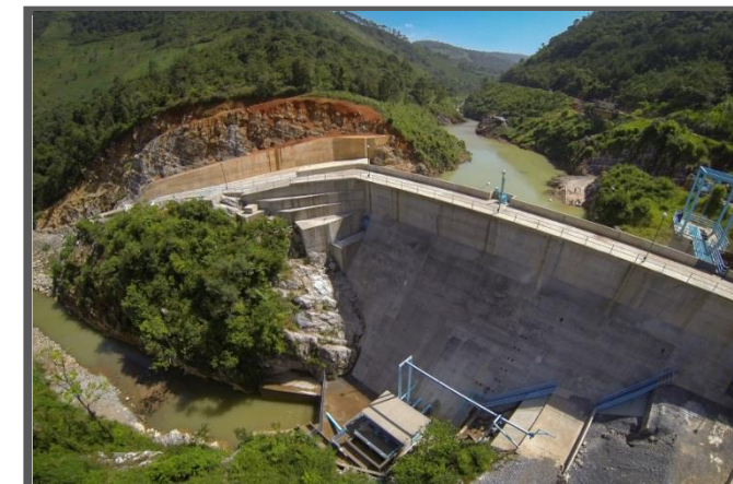
ELECTRICITY GENERATION MEXICO 46 MW
