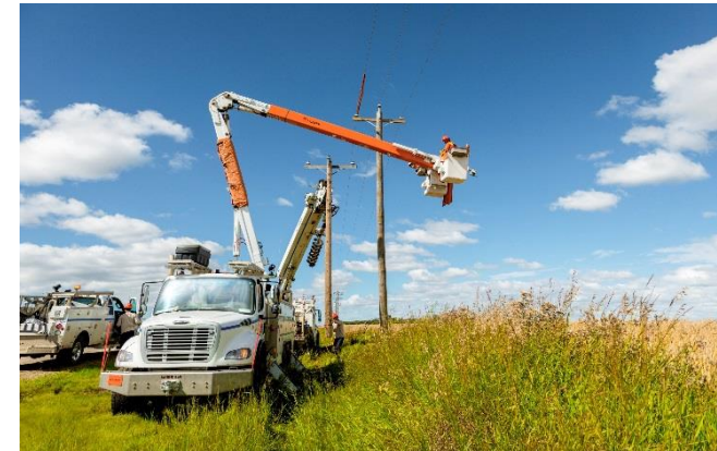
ELECTRIC DISTRIBUTION $2,476M Rate Base
