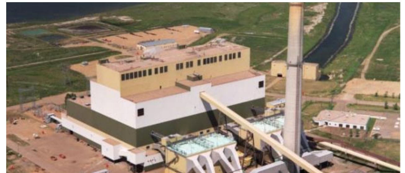
Sheerness Generating Station
