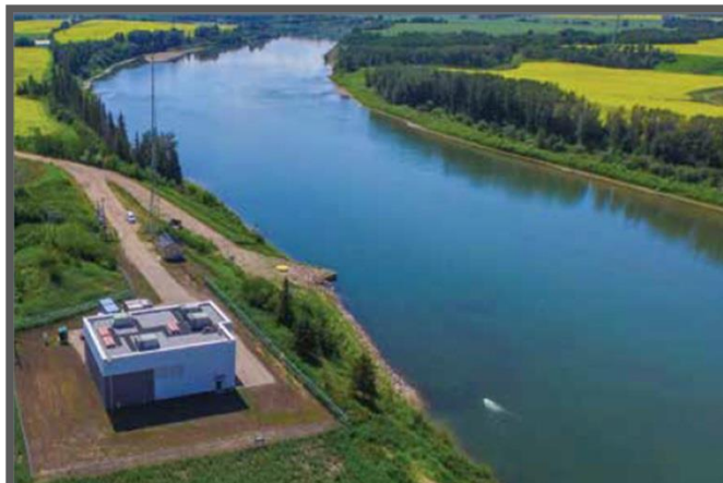
INDUSTRIAL WATER SERVICES CANADA 85,200 m 3 /day
