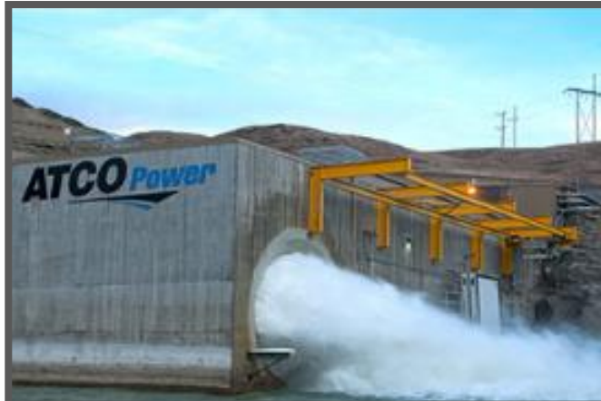
ELECTRICITY GENERATION CANADA 2,300 MW
