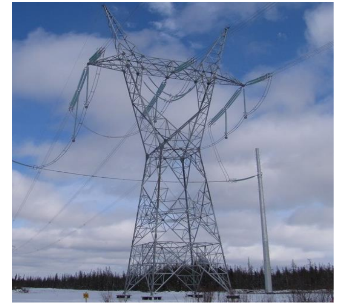
FORT MCMURRAY WEST 500 KV TRANSMISSION
