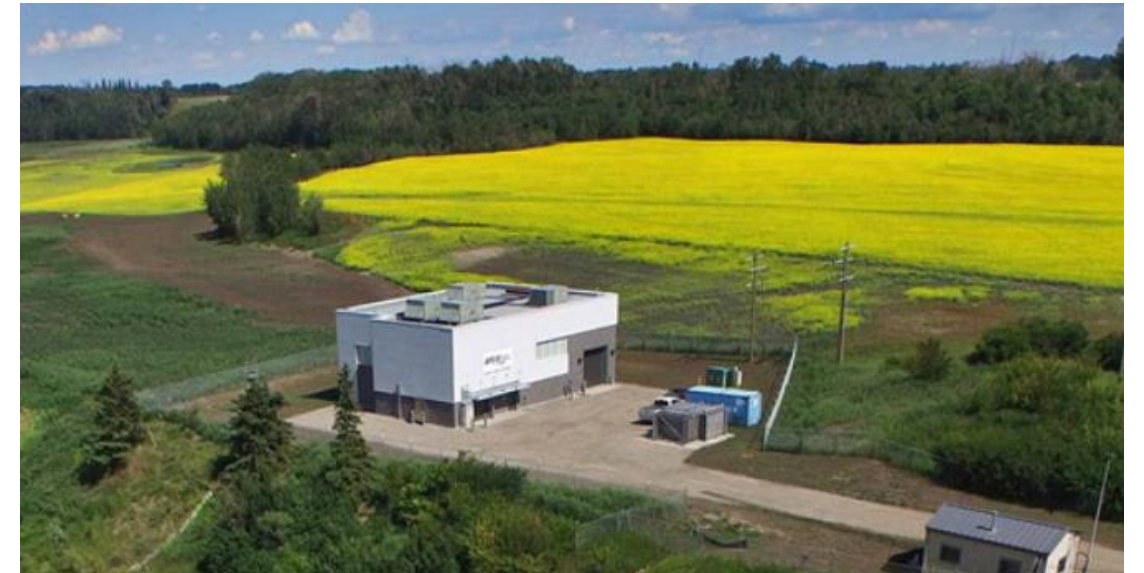
Heartland Industrial Water System
