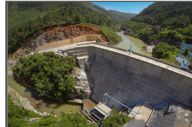
ELECTRICITY GENERATION MEXICO 46 MW
