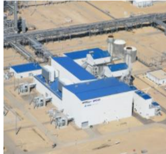
NATURAL GAS COGENERATION
