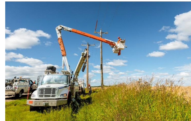
ELECTRIC DISTRIBUTION $2,476M Rate Base
