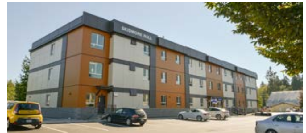
130-student dormitory Langley, Canada
