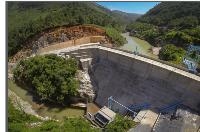
ELECTRICITY GENERATION MEXICO 46 MW
