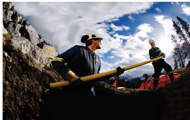
NATURAL GAS DISTRIBUTION $2,537M Rate Base
