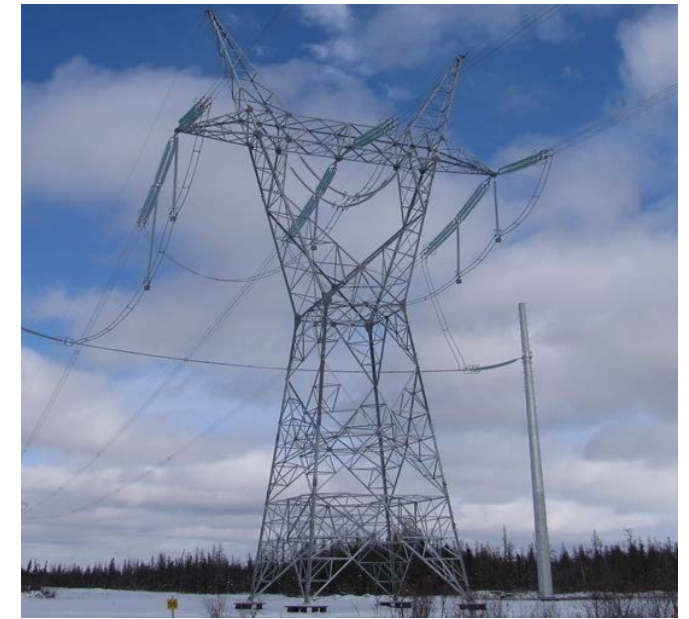
FORT MCMURRAY WEST 500 KV TRANSMISSION
