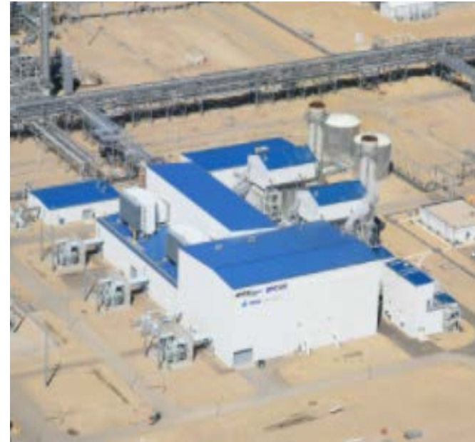
NATURAL GAS COGENERATION
