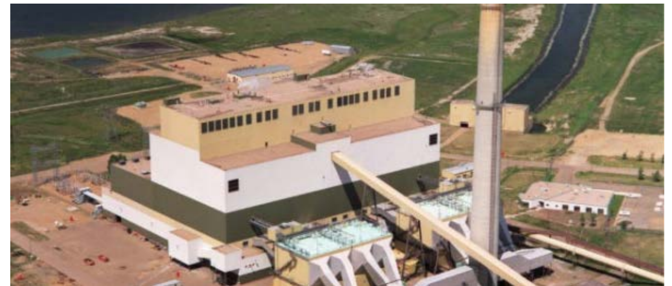
Sheerness Generating Station
