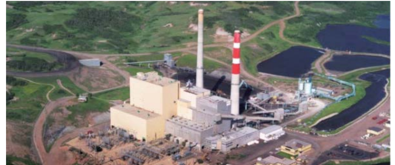
Battle River Generating Station
