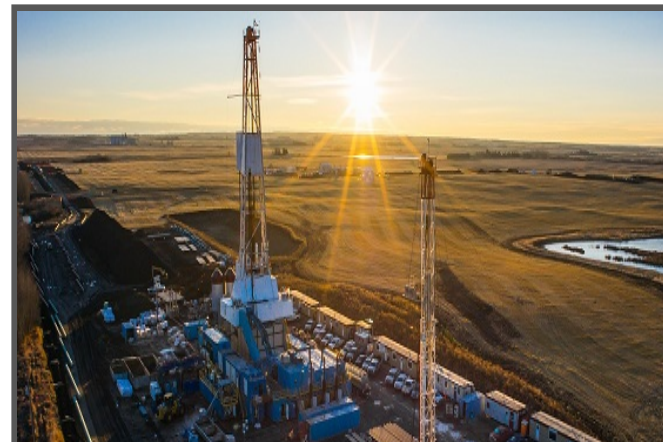
HYDROCARBON STORAGE CANADA 400,000 m 3
