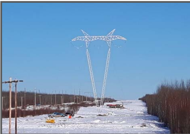
FORT MCMURRAY WEST 500 KV TRANSMISSION
