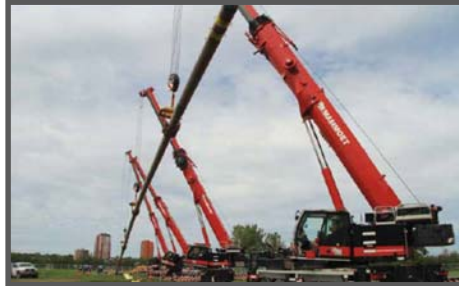
NATURAL GAS DISTRIBUTION
