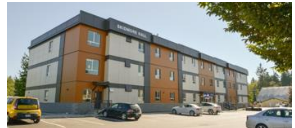
130-student dormitory Langley, Canada
