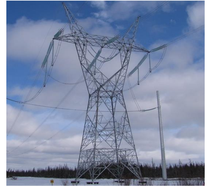
FORT MCMURRAY WEST 500 KV TRANSMISSION
