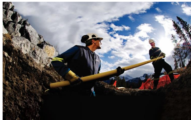
NATURAL GAS DISTRIBUTION $2,537M Rate Base
