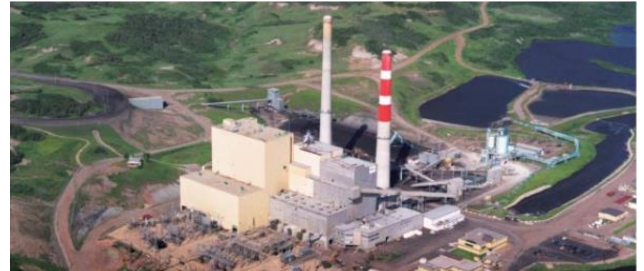
Battle River Generating Station
