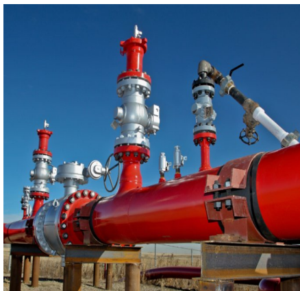
Natural Gas Pipeline Valve Assembly
