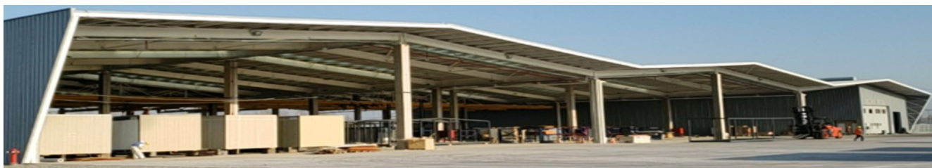
Chile Modular Structures Manufacturing Facility
