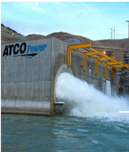
Oldman River Hydroelectric Plant
