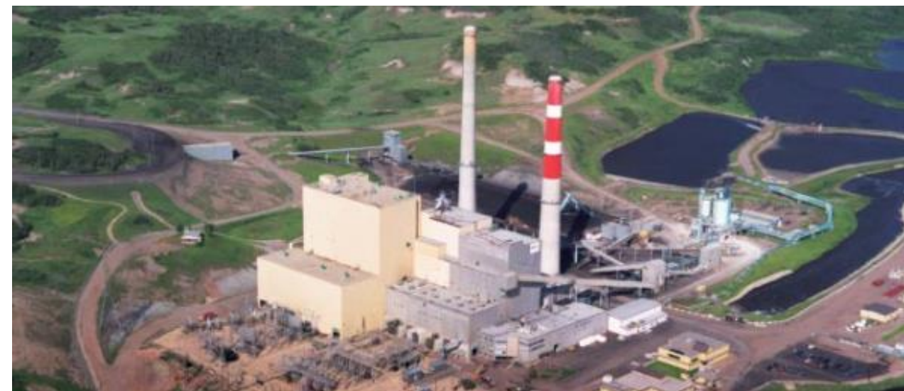
Battle River Generating Station
