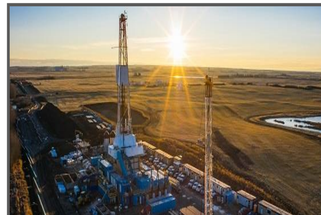
HYDROCARBON STORAGE CANADA 400,000 m 3
