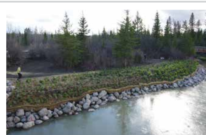
ATCO Pipelines completed remediation work on the Elbow River in Calgary, following a pipeline crossing exposure resulting from flooding in 2013. To ensure the safety and integrity of the pipeline, we covered the exposed pipe and rebuilt the riverbank to prevent future erosion.
