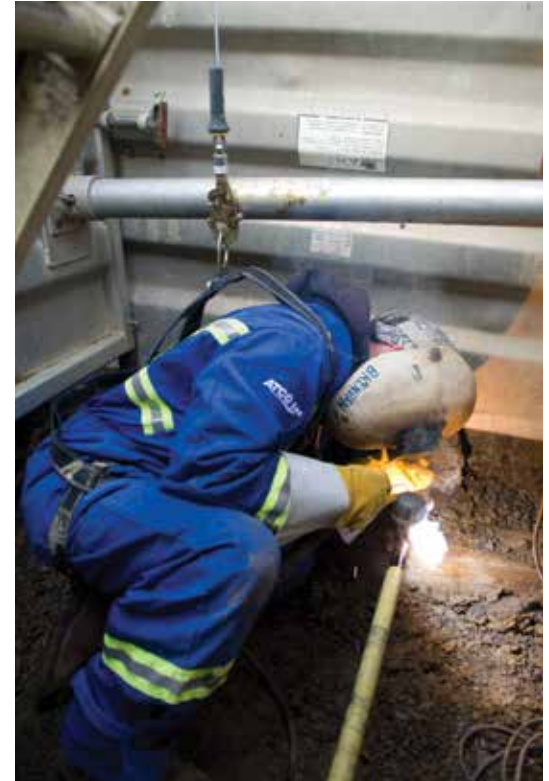
Brendan Walton, Pressure B Welder, ATCO Gas, uses an emergency trench rescue device while welding a stopper fitting onto a steel main. The device is used when employees are working in confined or restricted spaces enabling them to be quickly lifted to safety should the need arise.
