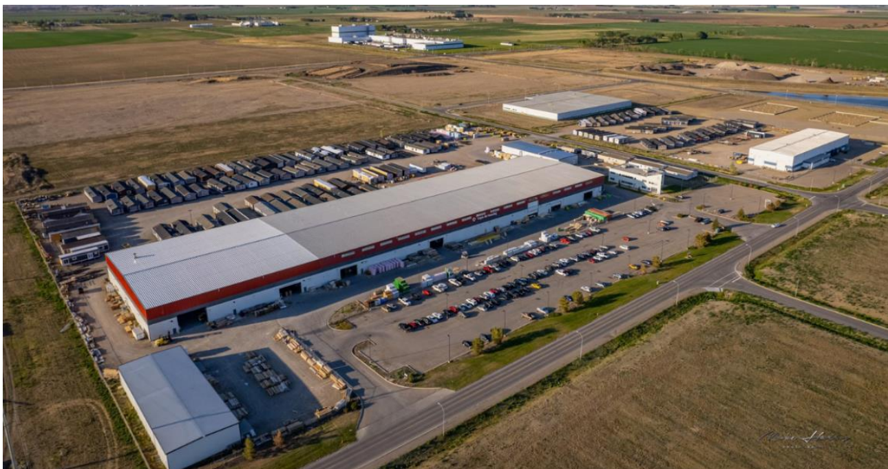
Triple M's 230,000 square foot manufacturing facility, Lethbridge, Alberta, Canada
