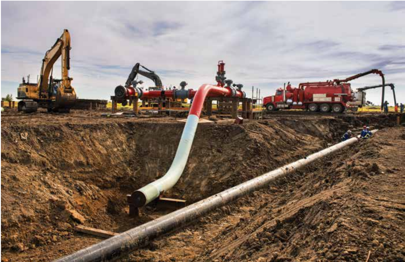
Construction crews installed 41 km of 508 mm (20 inch) pipeline in Norma, AB, to ensure sufficient supply of natural gas to meet growing demand in the Fort Saskatchewan and Edmonton regions.
