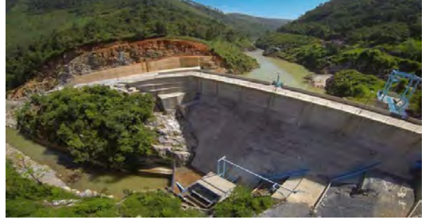
Hydroelectric power station, Veracruz, Mexico
