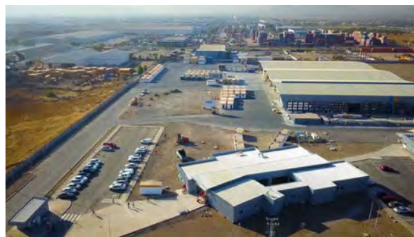
ATCO Sabinco, Manufacturing Facility, Santiago, Chile
