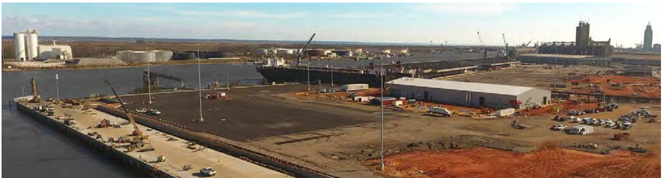
Construction Site of RoRo terminal, Mobile, Alabama
