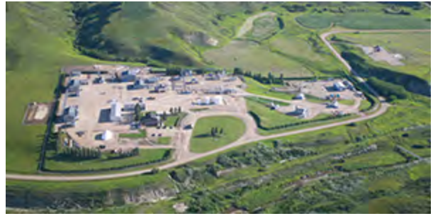
Natural gas storage facility, Carbon, Alberta
