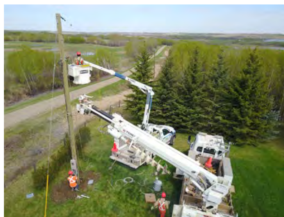
Electricity Distribution, Maintenance Work, Alberta
