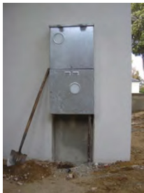
Conforming Installation (Recess Sealed from Cavity)
