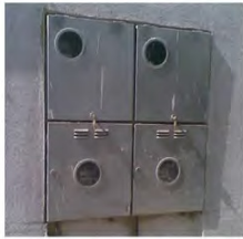
Figure 32 Gas Meter Box Viewing Apertures
