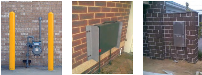
Figure 30 Gas Meter Box Protection (Examples)
