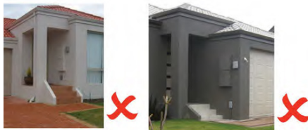
Figure 16 Gas Meter Box Installed Above Flight of Stairs (Unacceptable Positions)
