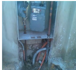
Non-Conforming Installation (Other Services Installed)
