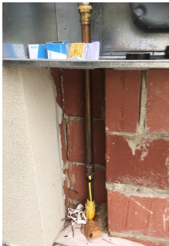
Non-conforming Installation (Surface is not finished, not sealed, and cracks in the brickwork, which provide a leak path to the cavity)
