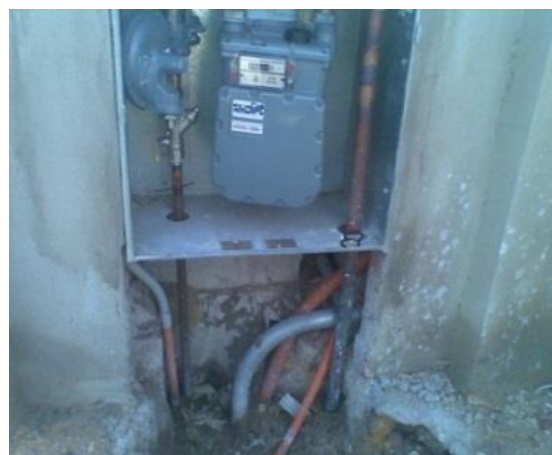
Non-conforming Installation (Other Services Installed)
