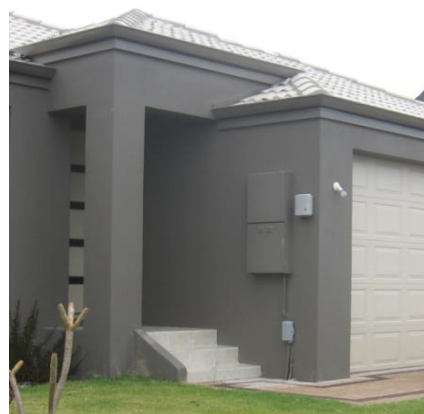
Figure 23: Gas Meter Box Installed Above Flight of Stairs (Unacceptable Positions)
