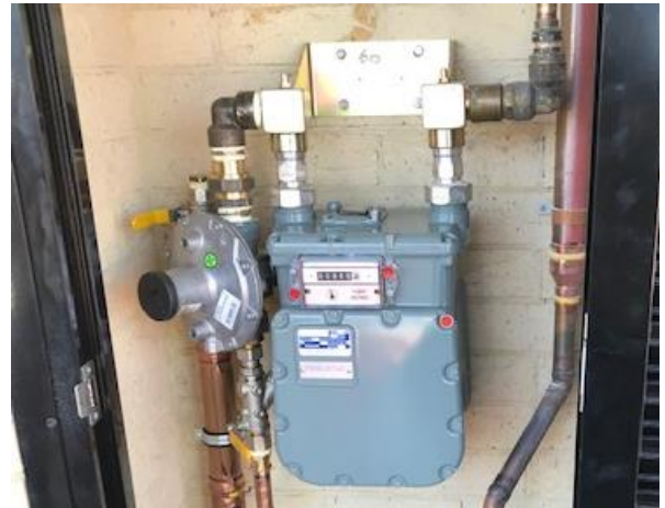
Right: AL12/AL18 Meter Bracket
