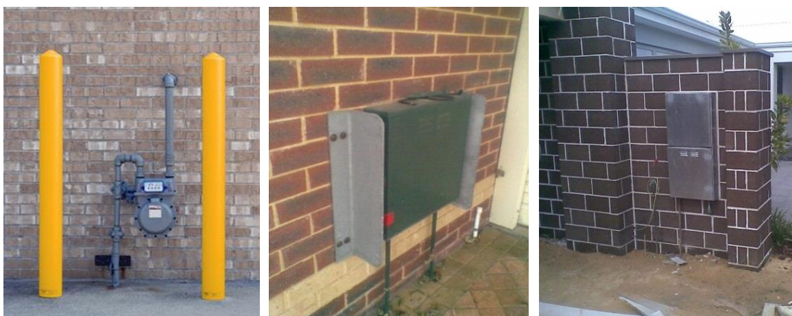
Figure 46: Gas Meter Box Protection (Examples)
