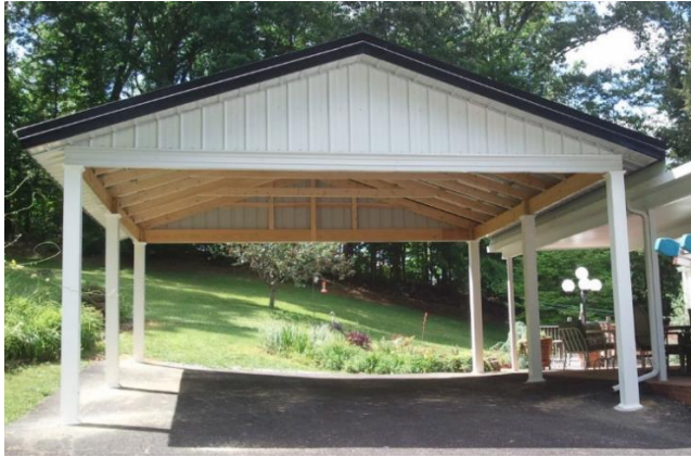
Acceptable – Service Line is Ventilated
