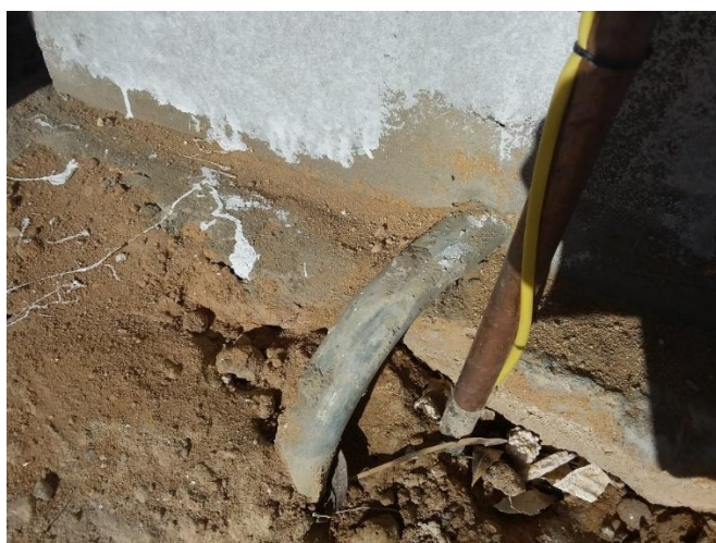
Figure 22: Non-compliant Service Separation (Less than 150 mm)
