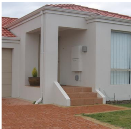
Figure 23: Gas Meter Box Installed Above Flight of Stairs (Unacceptable Positions)
