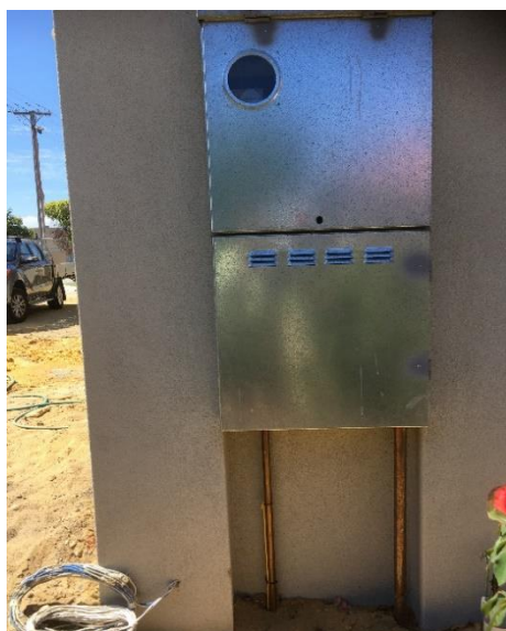
Conforming Installation (Recess Sealed from Cavity)
