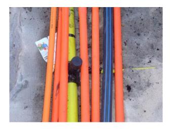
Figure 5 Unacceptable Open Trench (encroaching utilities)
