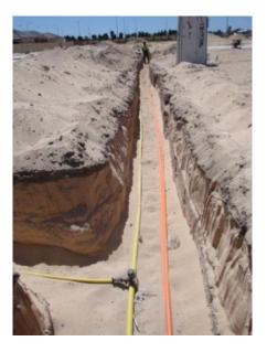
Figure 4 Acceptable Open Trench - Example
