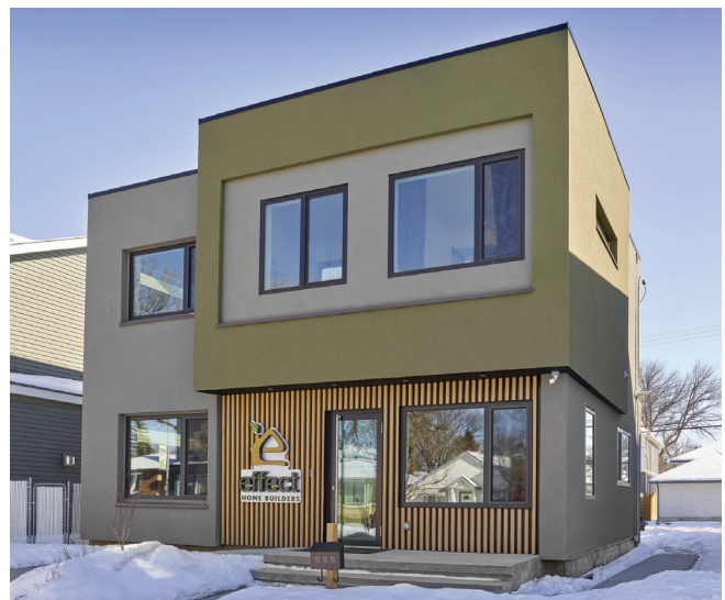
The Effect Home Builders Office in Edmonton, Alberta is the first office building in the city to be disconnected from the electrical grid. The building uses a solar PV system, mCHP units, battery storage and an advanced HP+ wall system. (ATCO, Effect Home Builders and NGIF)
