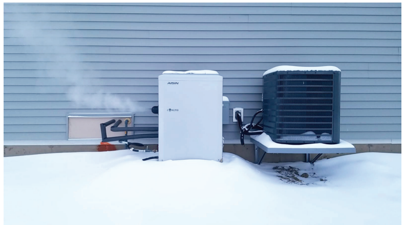
Brookfield Residential's Low Carbon Discovery Home with mCHP integration into the home heating system. (Top photo: Edmonton Journal; Bottom photo: ATCO)
