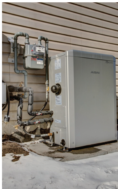
mCHP integration into a home heating system (left) and a mCHP retrofit in an urban home (right). (ATCO)
