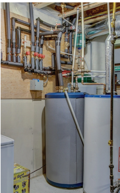
mCHP integration into a home heating system (left) and a mCHP retrofit in an urban home (right). (ATCO)
