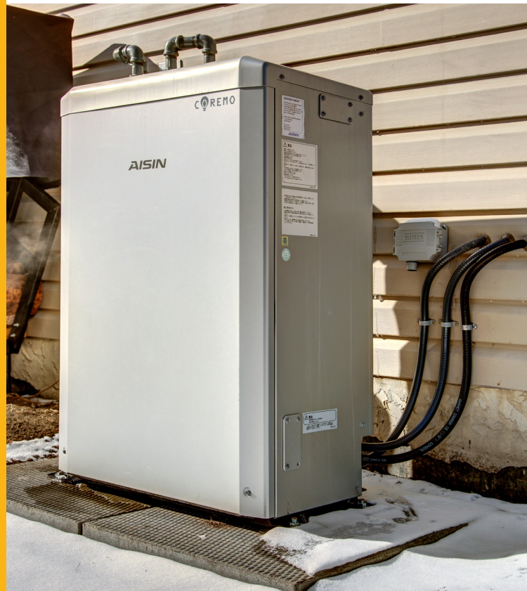
AISIN 1.5kW mCHP system.
