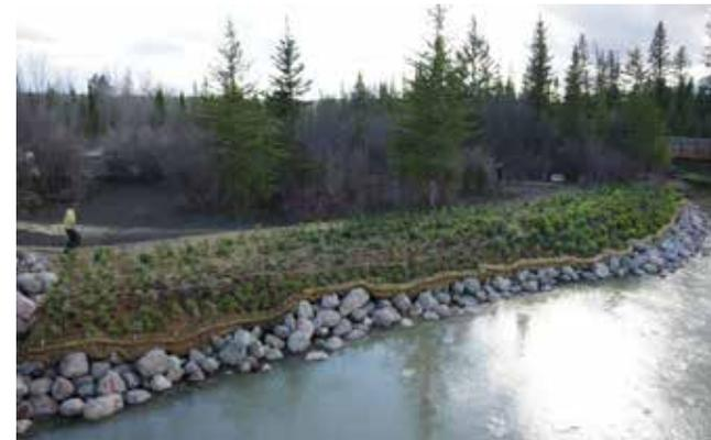
ATCO Pipelines completed remediation work on the Elbow River in Calgary, following a pipeline crossing exposure resulting from flooding in 2013. To ensure the safety and integrity of the pipeline, we covered the exposed pipe and rebuilt the riverbank to prevent future erosion.
