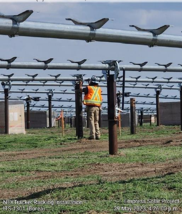
Solar Array of Piles and Racking
