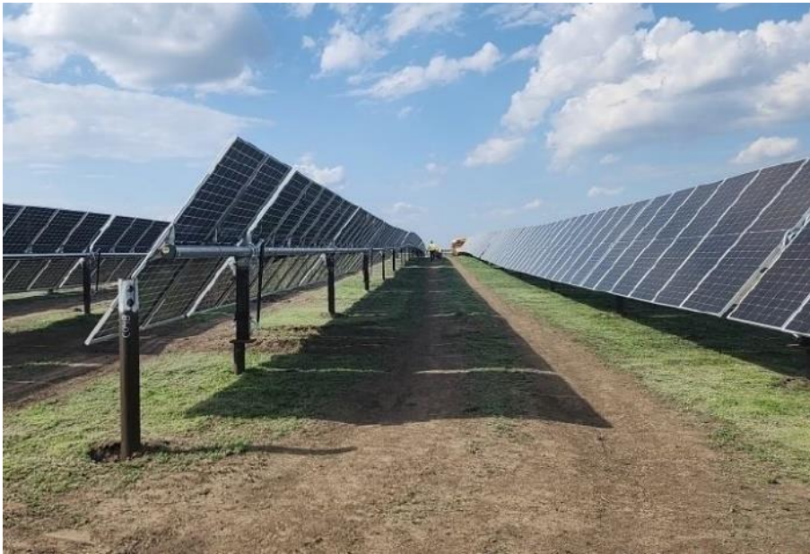
Solar Panels Installed on Racking and Piles
