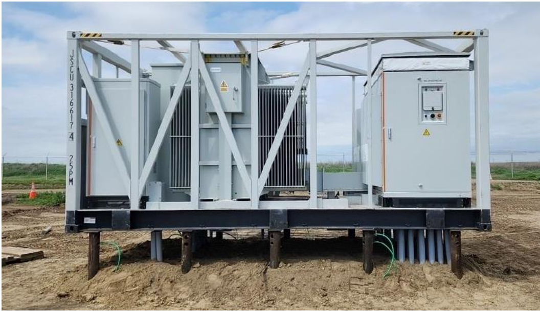
Inverter / Transformer Unit Installed on Piles
