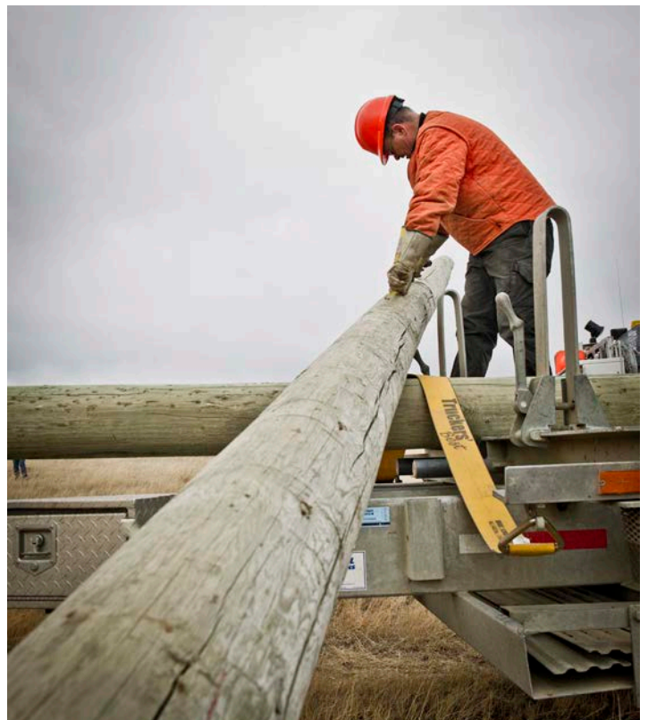
Unloading structures from trailer
